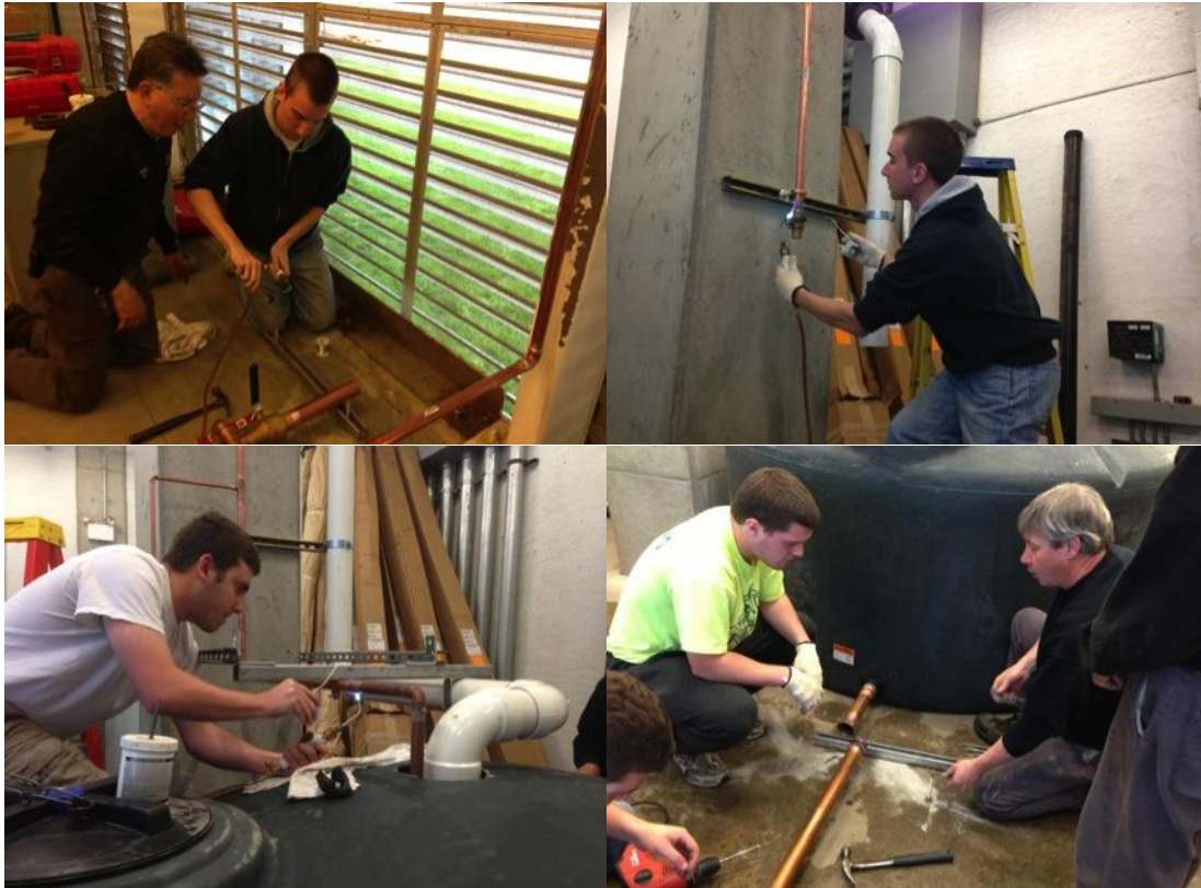
FIGURE 7 (continued) THE FINAL PRODUCT AND TESTING
